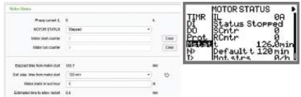
Figure 77 - Motor status via Easergy Pro and local panel
